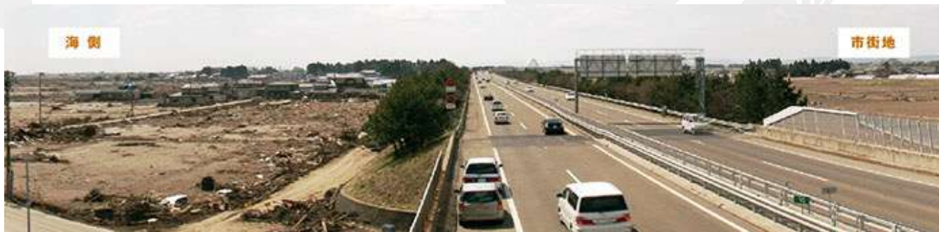
仙台東部道路が内陸の市街地への津波・がれきの流入を抑制 The Sendai-Tobu Road blocked the tsunami and rubble from reaching farther inland.
